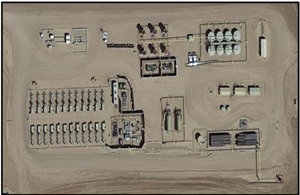
2020 Design (6 oil tanks)
